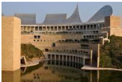
Fig 3.7, Exterior view of the museum
