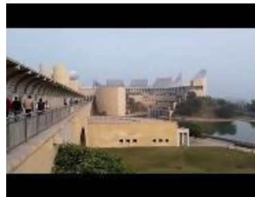
Fig 3.8, Bridge connecting Complex A
