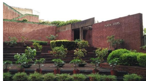
Fig 2.33 Use of brick with greenery
