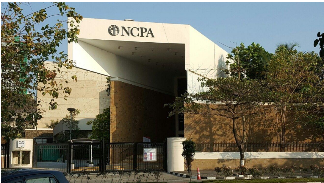
Fig 2.38 View of the front side
