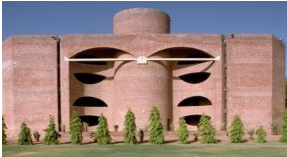
Fig 2.2.7 : View of Faculty Block
