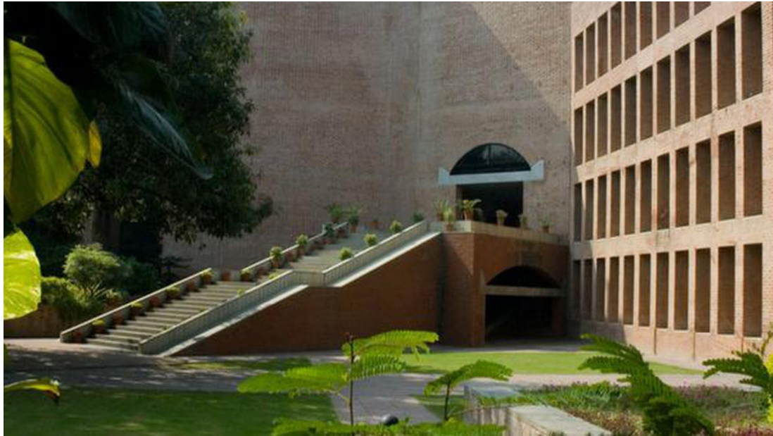
Fig 2.2.2 : Entrance to the Building
