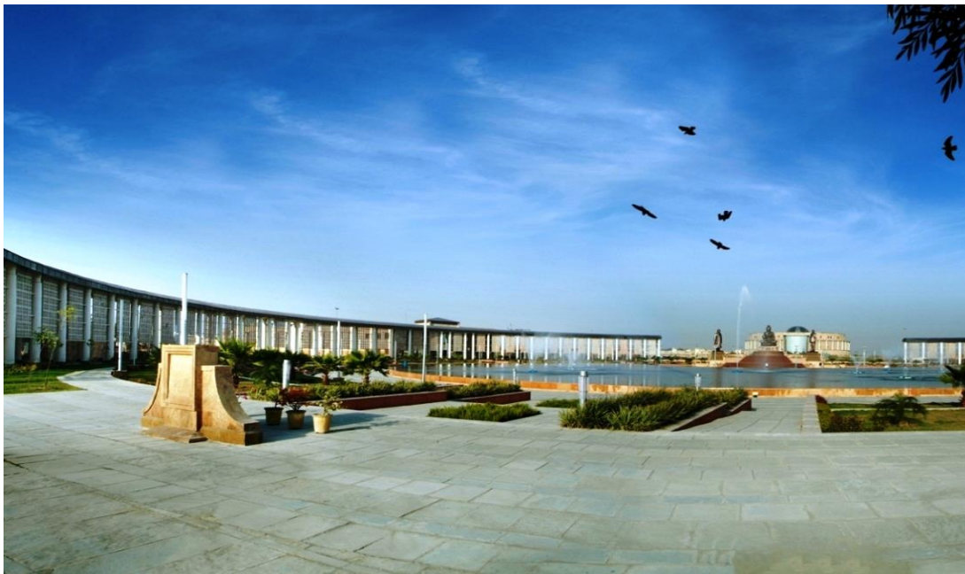
Fig 2.1.2 : View from the front side
