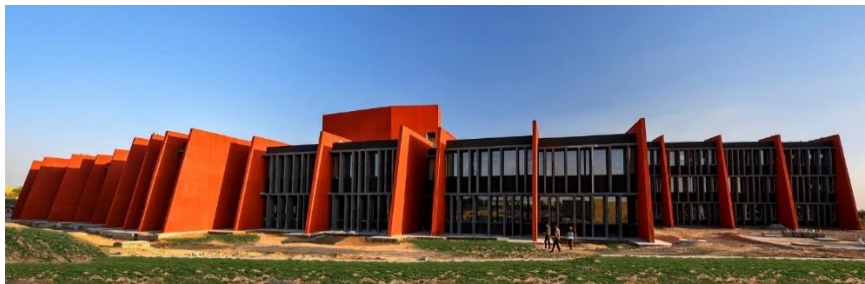
Fig 3.7 View of the school
