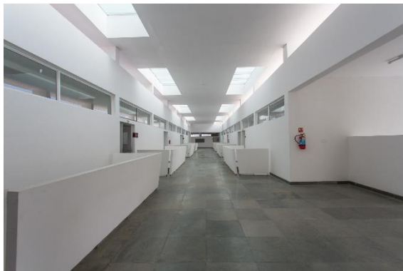
Fig.3.16 Skylight in the corridors
