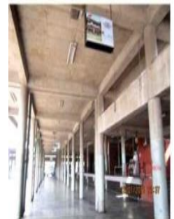
COLUMN & BEAM STRUCTURE
