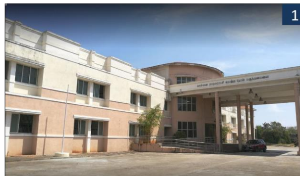
Figure 2.3.4: front view admin block
