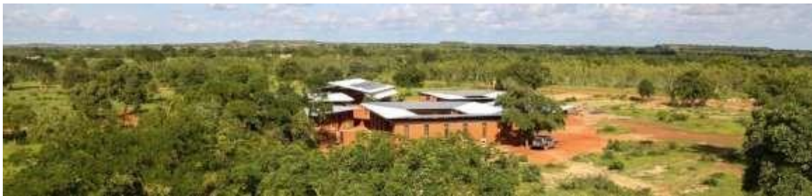
Figure 3. 16 Noomdo orphanage site view
