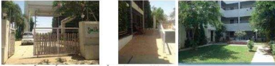
Figure 3. 11 Entrance and courtyard
