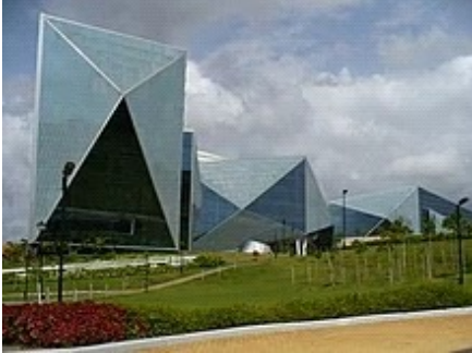
The Development Centre in campus
