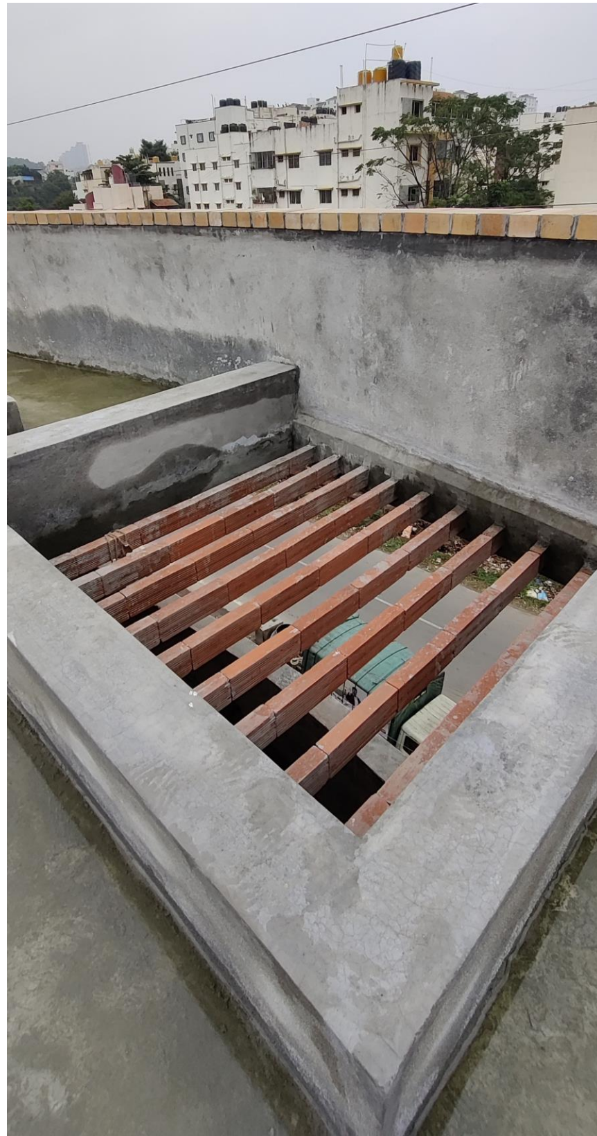
Pergolas made of terracotta clay blocks With reinforcements welded to metal frame.
