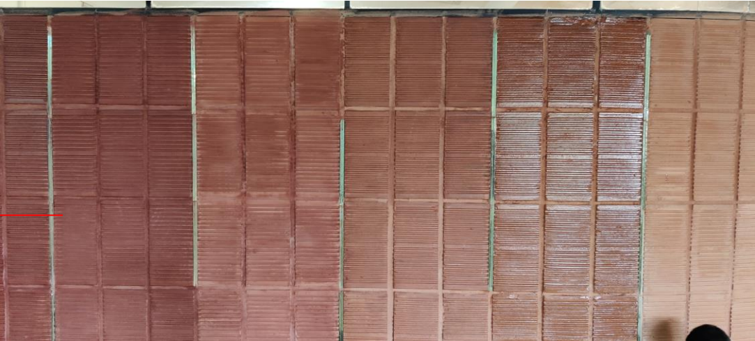
Sample for different types of lacquer polish finishes on the Basement office wall.
