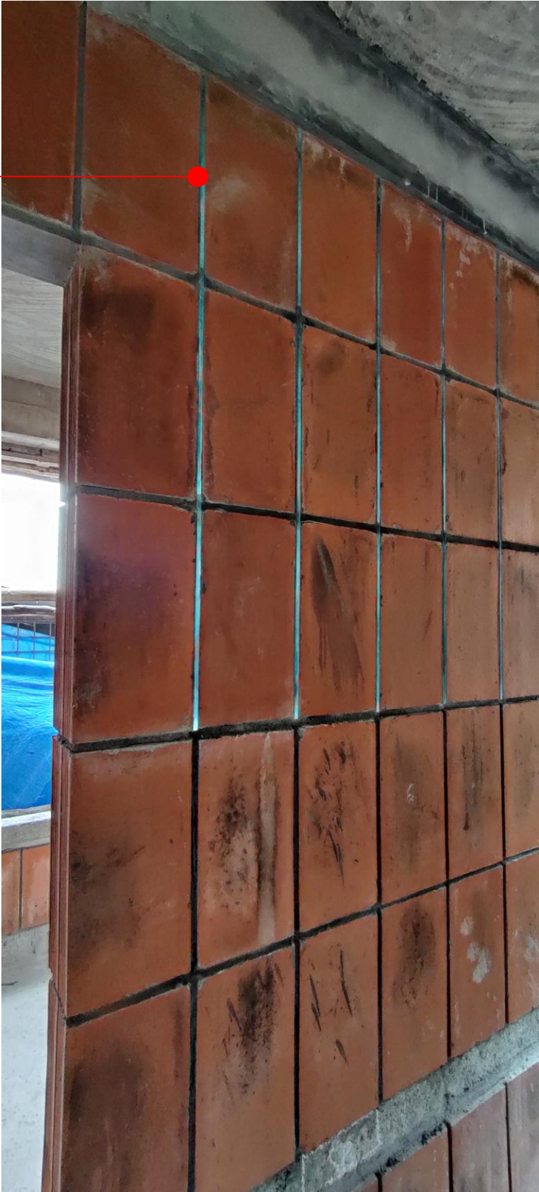
Utility Partition Wall
