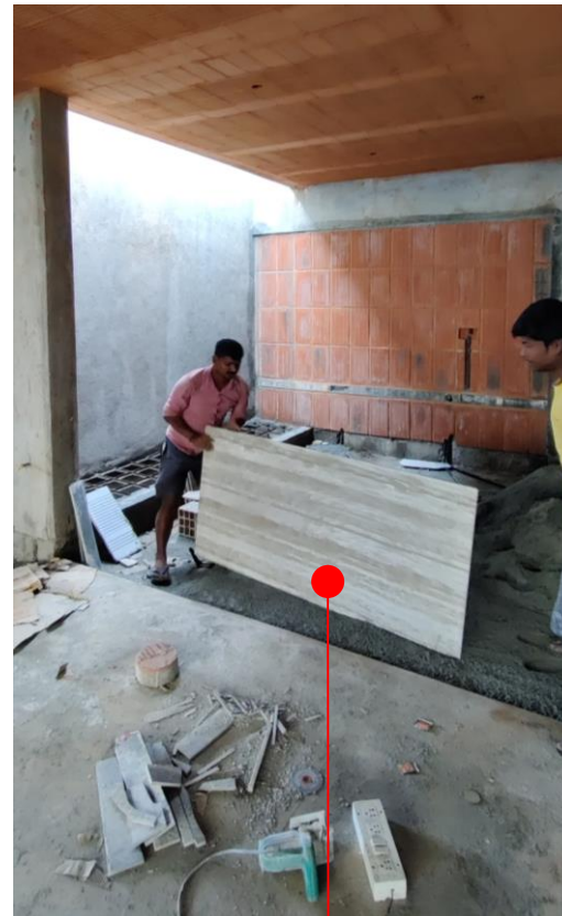
Laying of Jaisalmer Stone flooring
