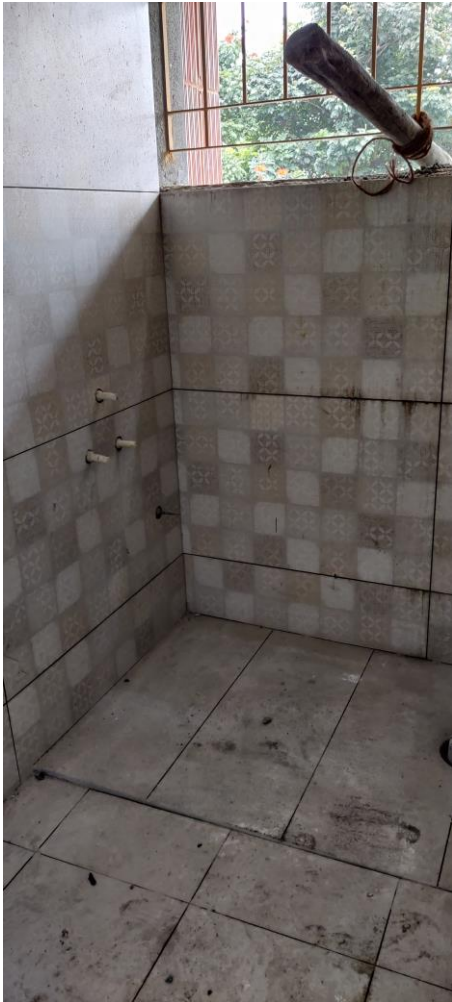
Sadarahalli stone for The Bath area
