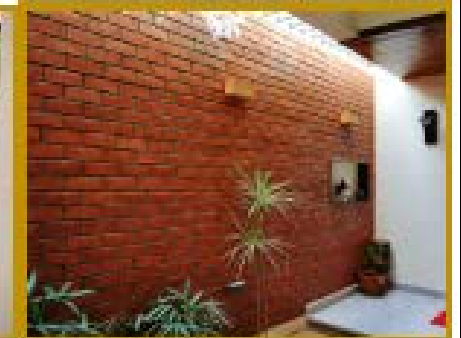
Exposed Brick Wall
