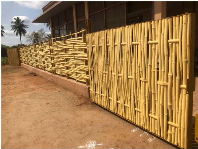
Painted using epoxy paint to prevent from termites or insects and climate.
