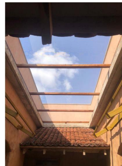
Skylight with slope roof (terracotta)
