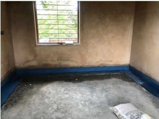
Oxide skirting and border (patti)
