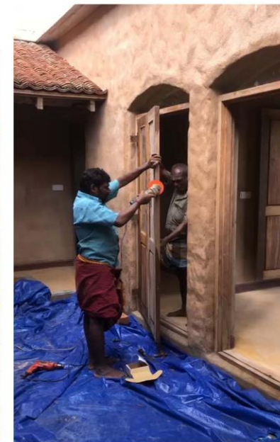
On site carpentring work, with Kali marudhi wood, palakatu vengai wood (available only in kerala)
