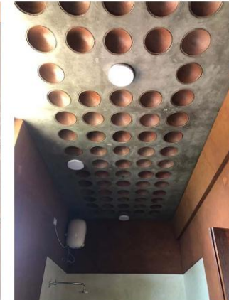
Fillers slab throughout the house
