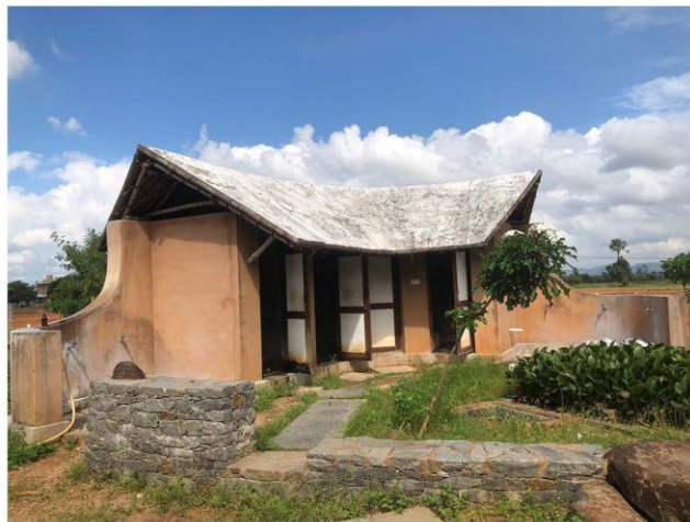
Bathroom with CSEB walls and mud plaster finish, landscape with random rubble and tandoor stone.
