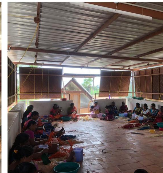
Bamboo blinds covered for restricting heat and excess light.
