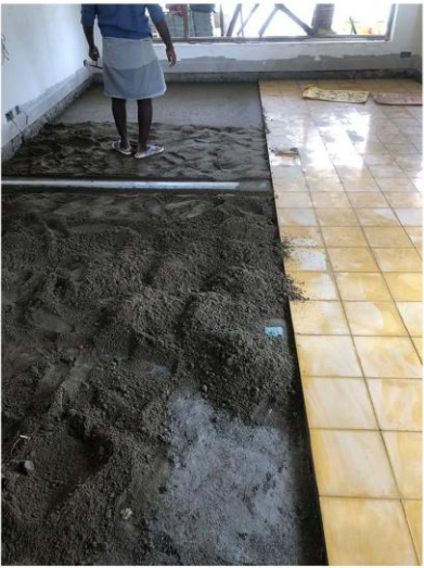
Marking and laying of Athangudi tiles by skilled men from Karaikudi.
