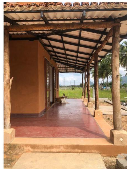
Raw wooden tree logs used as pillars on stone base.
