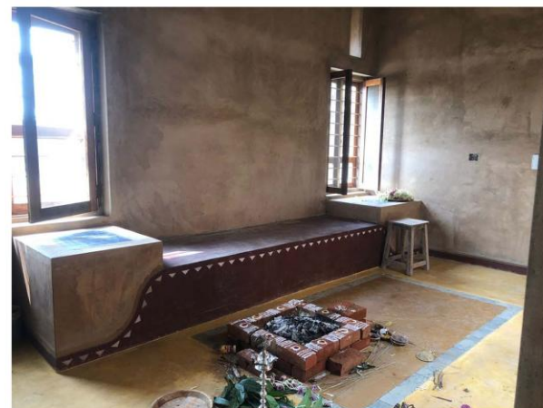
Living area- oxide flooring, mud plastering walls and thinnai concept.
