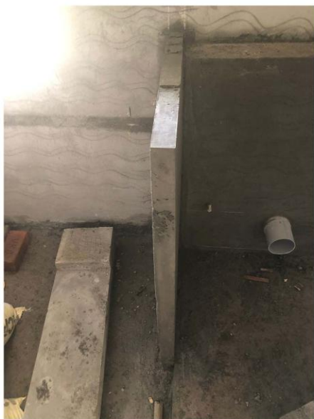
Half/ dwarf wall and wash basin counter on-site casting
