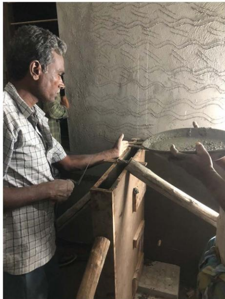
Half/ dwarf wall and wash basin counter on-site casting
