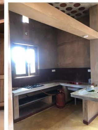
Fillers slab ceiling, on-site casted exposed concrete counter top and mud plastered walls.
