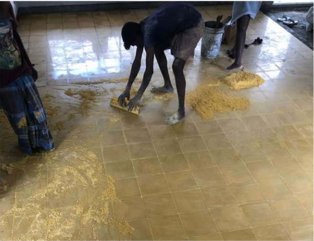
Gaps filling after 3 days from laying using oxide powder with white cement.
