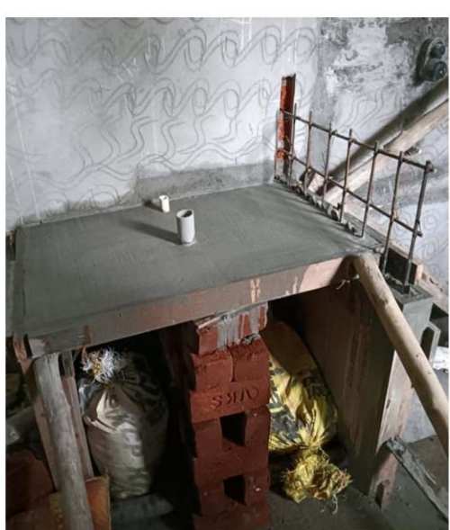
Half/ dwarf wall and wash basin counter on-site casting
