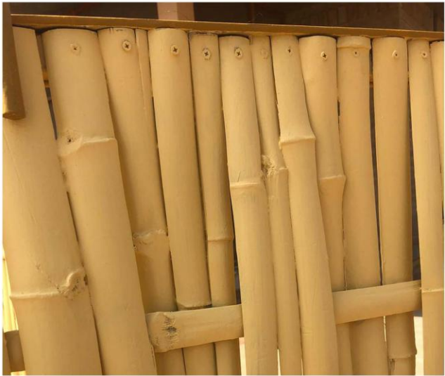
Painted using epoxy paint to prevent from termites or insects and climate.
