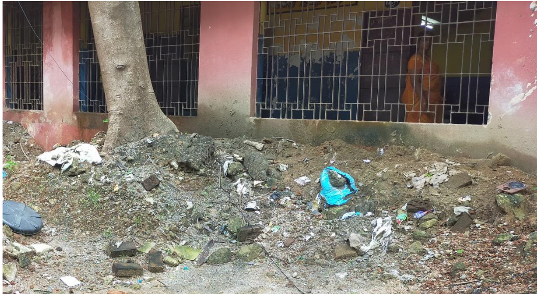
Debris in the site
