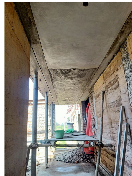
Oxide finishing in roof
