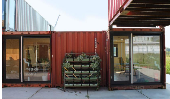
Fig 4.3 No foundation piles
