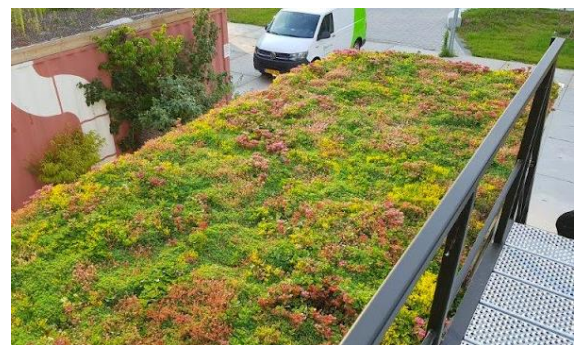
Fig 4.7 Green roof as insulation
