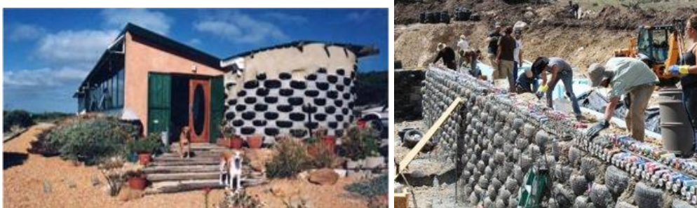
Fig 09 – Construction using upcycled material
