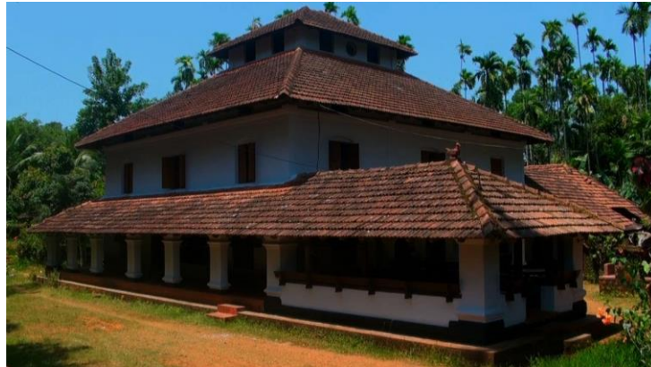
Fig 2.6 Traditional building of Kerala
