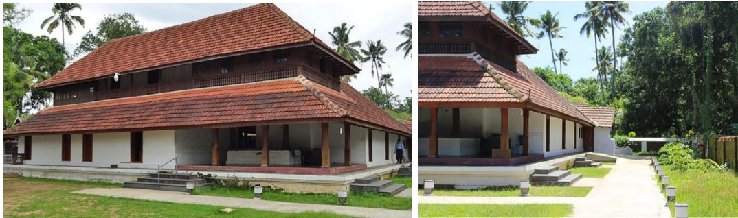
Fig 3.10 Front view and Verandah
