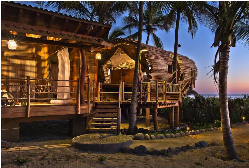
Fig 3.49 Image showing Tree house Suite, Mexico
