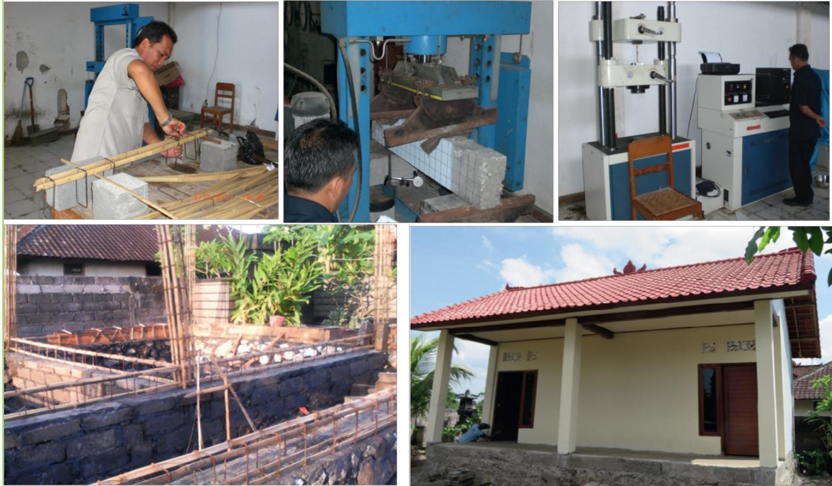
Fig 8.1 Construction process of Bamboo reinforcement structure
