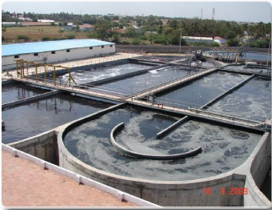
Fig 2.1 Nine traditional common effluent treatment plants (ETP)
