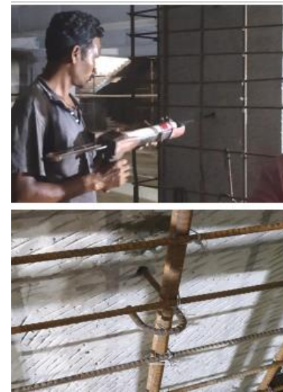
Drilling of Column – hook fixing .
