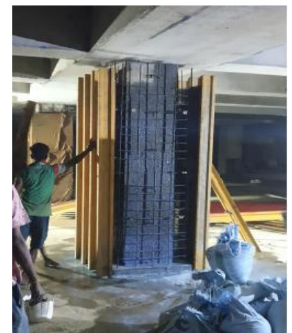
Fixing of shutters
