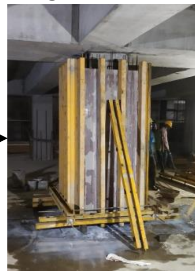
Removal of shuttering
