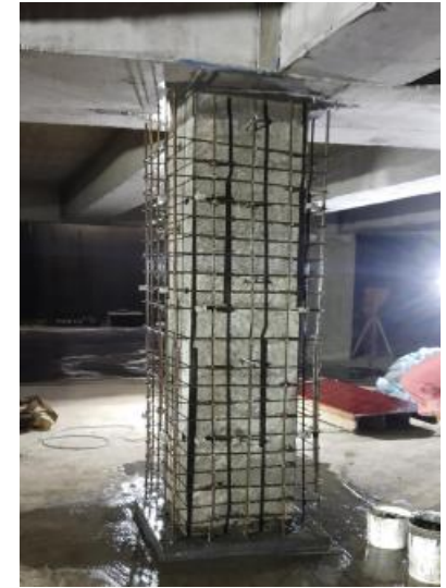
Concreting of column starter
