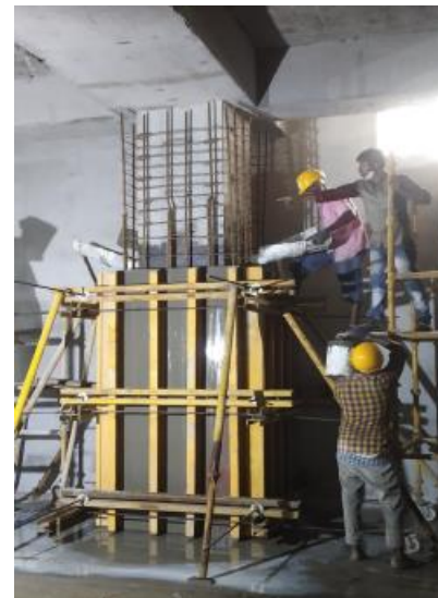
Removal of shuttering after 12 hours
