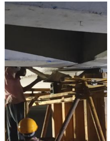
Facilitating microcrete pouring from the top
