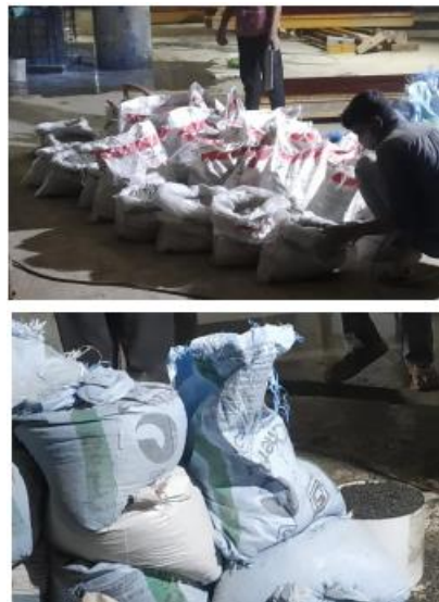
Materials for Microcrete - Fosrac Renderoc RG, 8 - 10 mm of Aggregates & water
