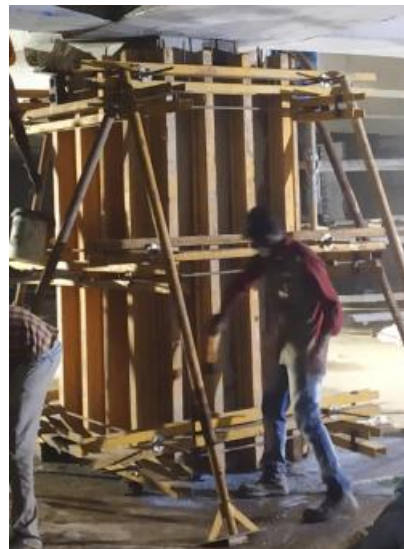
Compaction using wooden hammer
