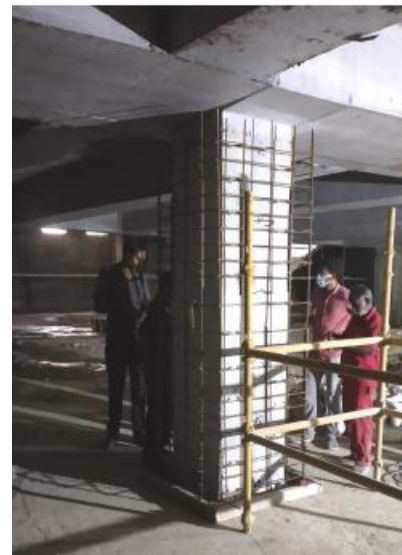
Placing of reinforcement
