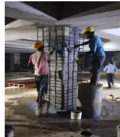
Applying of Fosroc Nitobond bonding agent using brush
