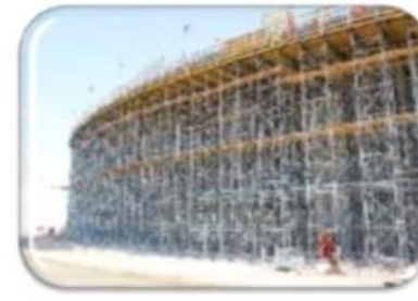
PMV and Formwork yard
