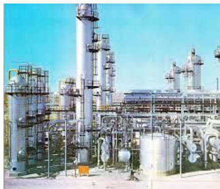
Fig 3.1 Bidboland Gas treating plant
