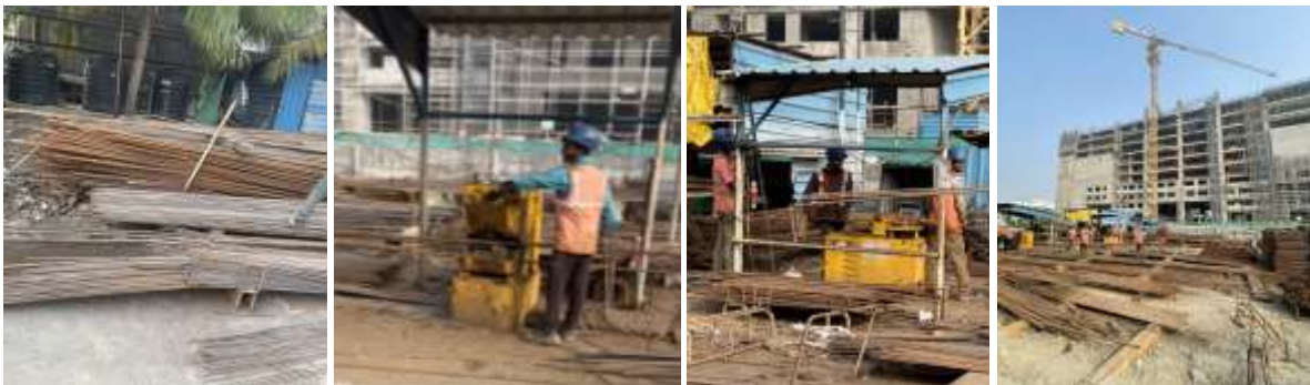
Fig 4.4 Site Images – Rebar process
