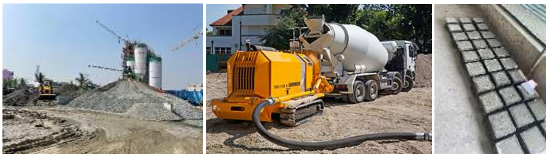
Fig 4.8 Site Images – Concreting
