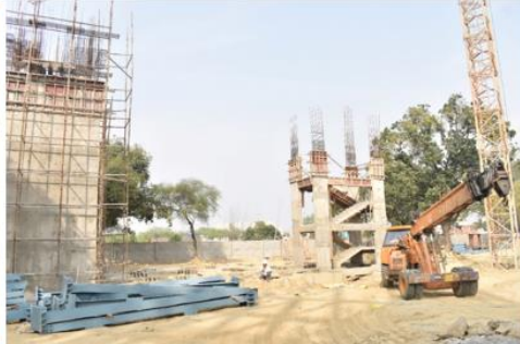
Staircase Core on progress
