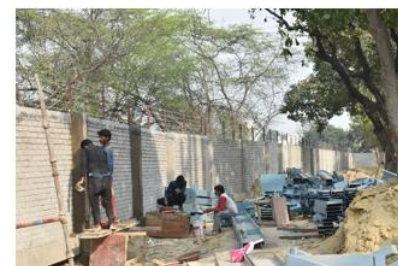
BOUNDARY WALL BRICK WOKR IN PROGRESS
