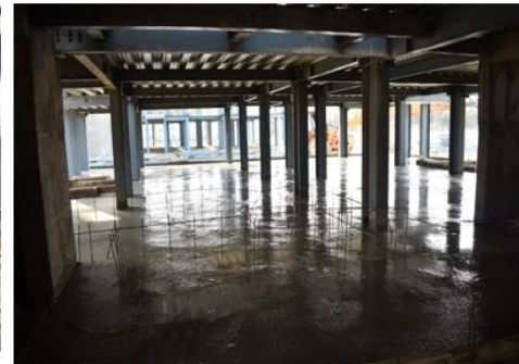
Stilt floor Concreting
