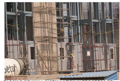
BLOCK C SIP WALL INSTALLATION IN PROGRESS OF FIRST FLOOR
