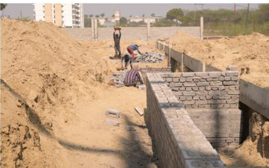
COMMUNITY CENTER PLINTH BEA, CASTING DONE AND SOIL FILLING IN PROGRESS
