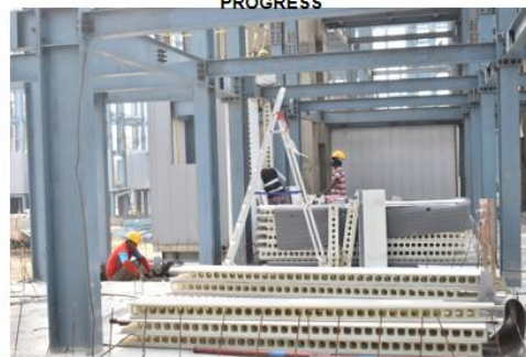
1 ST FLOOR & 2 ND Floor PANEL WORK ON PROGRESS
