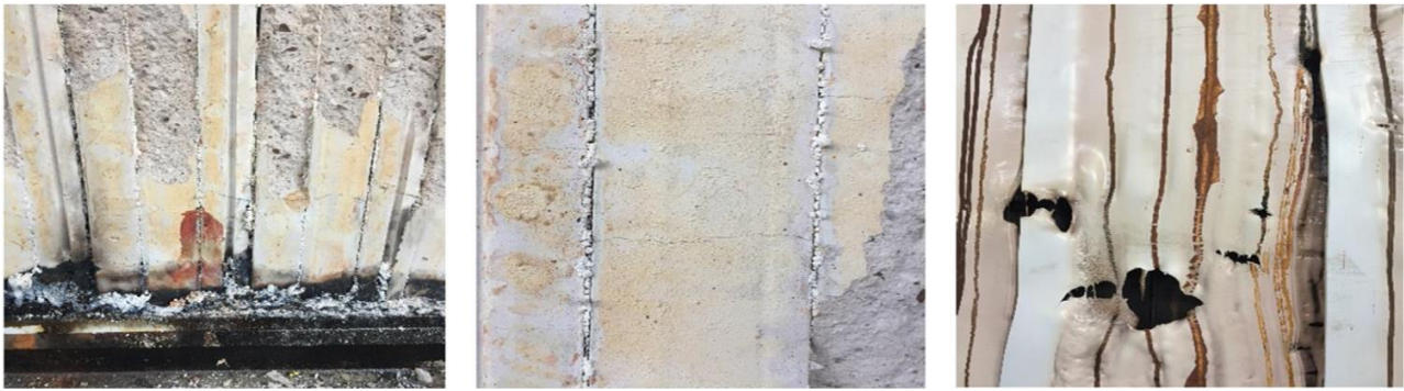
Fig 2.6.1b Details of the final aspect of the concrete's surfaces.
