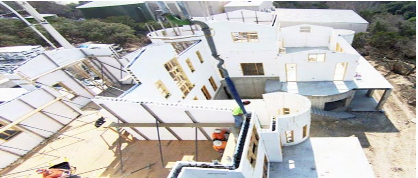
Fig 2.1.a Stay- in – place Formwork system
