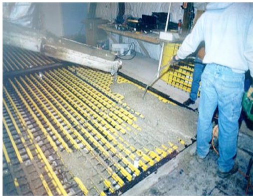
Fig. 4.14: FRP concrete deck preparation
