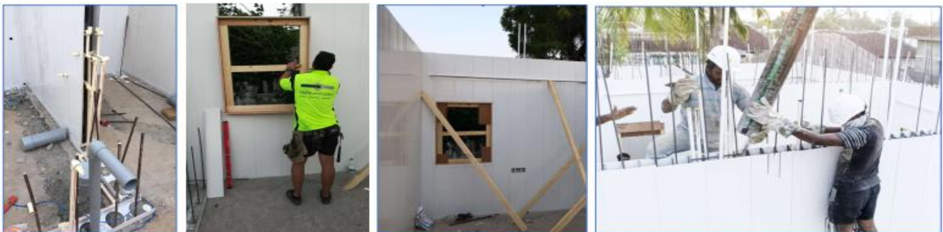
. Fig 2.5.7.C.2 DOORS, WINDOWS AND CONCRETING
