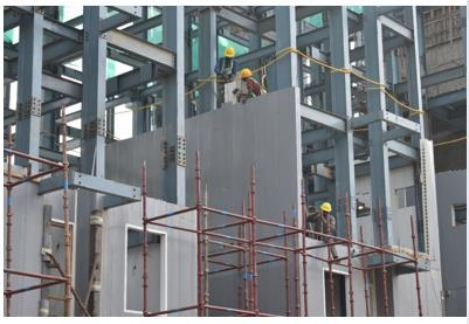
BLOCK C SIP WALL INSTALLATION IN PROGRESS OF FIRST FLOOR
