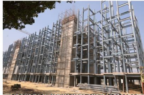
BLOCK D SIP WALL INSTALLATION IN PROGRESS OF FIRST FLOOR AND PEB ERECTION OF THIRD PHASE IN PROGRESS
