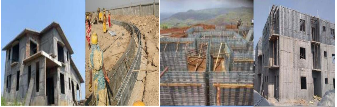
Fig 1.2 Structural stay- in – place Formwork system
