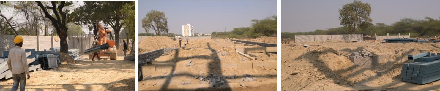
COMMUNITY CENTER PLINTH BEAM CASTING DONE AND SOIL FILLING IN PROGRESS
