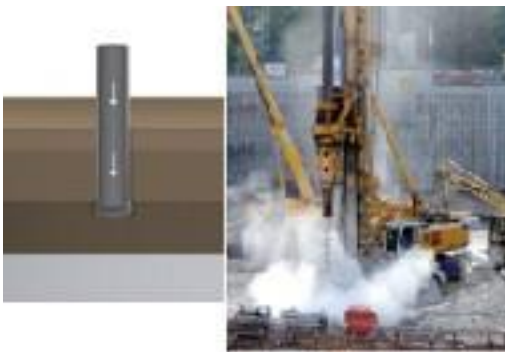
Figure 66 : Boring for pile
