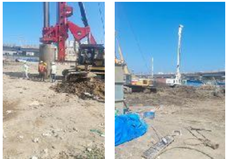
Figure 69 : Pile riggers in the site
