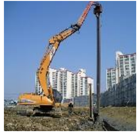
Figure 29 : Driven Pile
