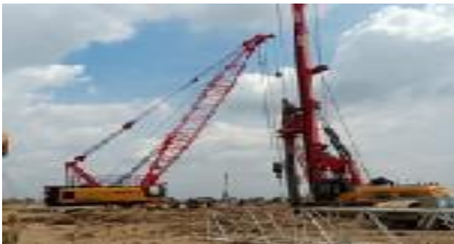
Figure 79 : Equipment in the site
