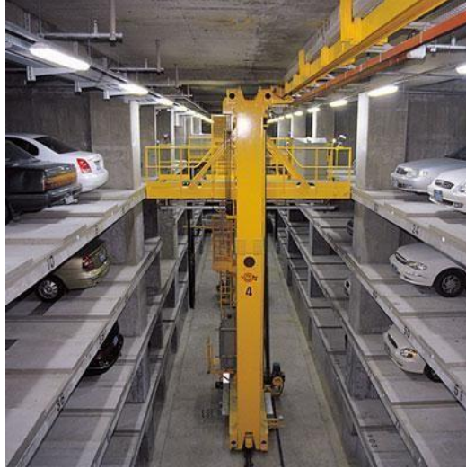
Figure 1.1: Integrated car parking solution
