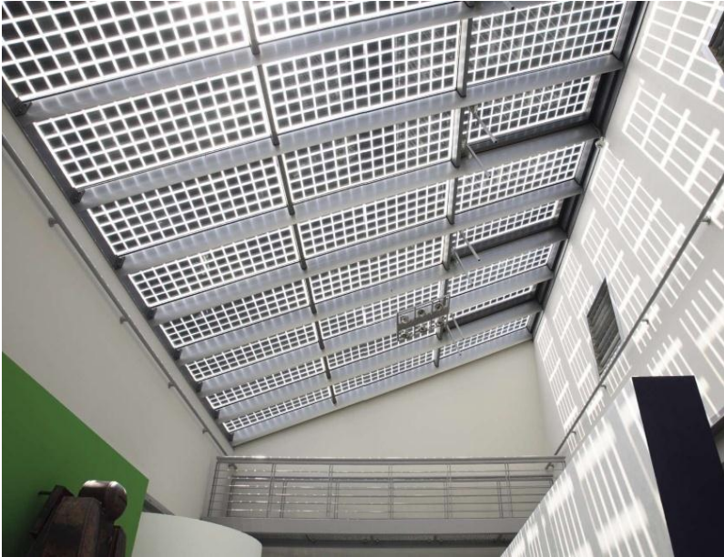
FIG. Showing Building Integrated Photo Voltaic
