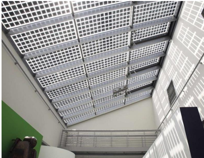
FIG. Showing Building Integrated Photo Voltaic
