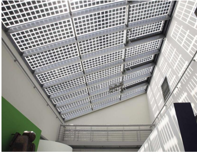
FIG. Showing Building Integrated Photo Voltaic
