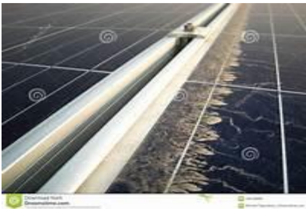
Soiling, such as dust, on PV modules reduces power output.
