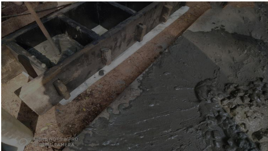
Fig:3.13 Casting the compression cubes
