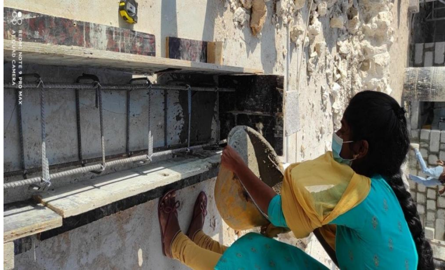
Fig :3.16 casting of beam
