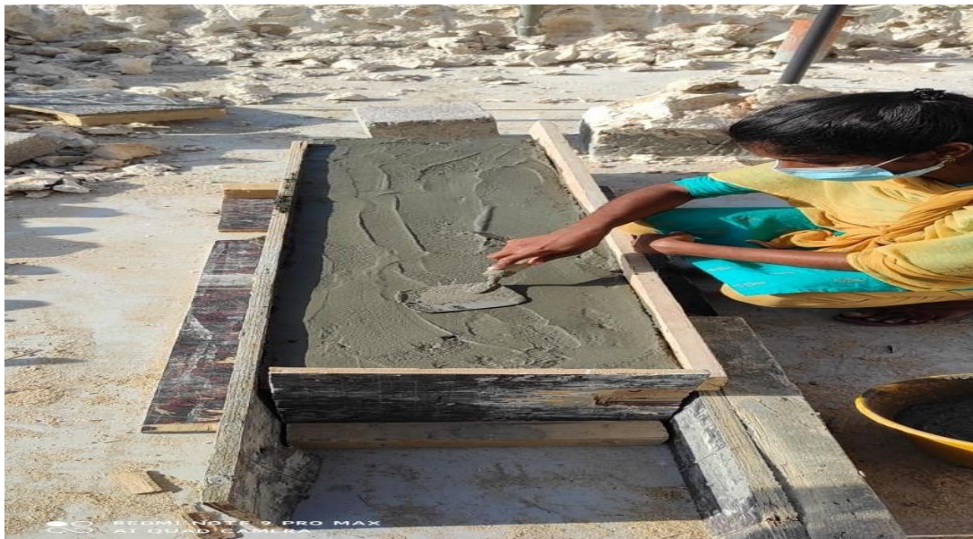
Fig:3.17 Compacting the concrete beams
