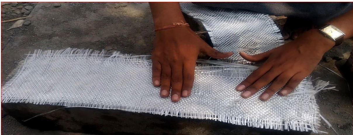
Fig:3.22 GFRP wrapped 3 layers in RC beams
