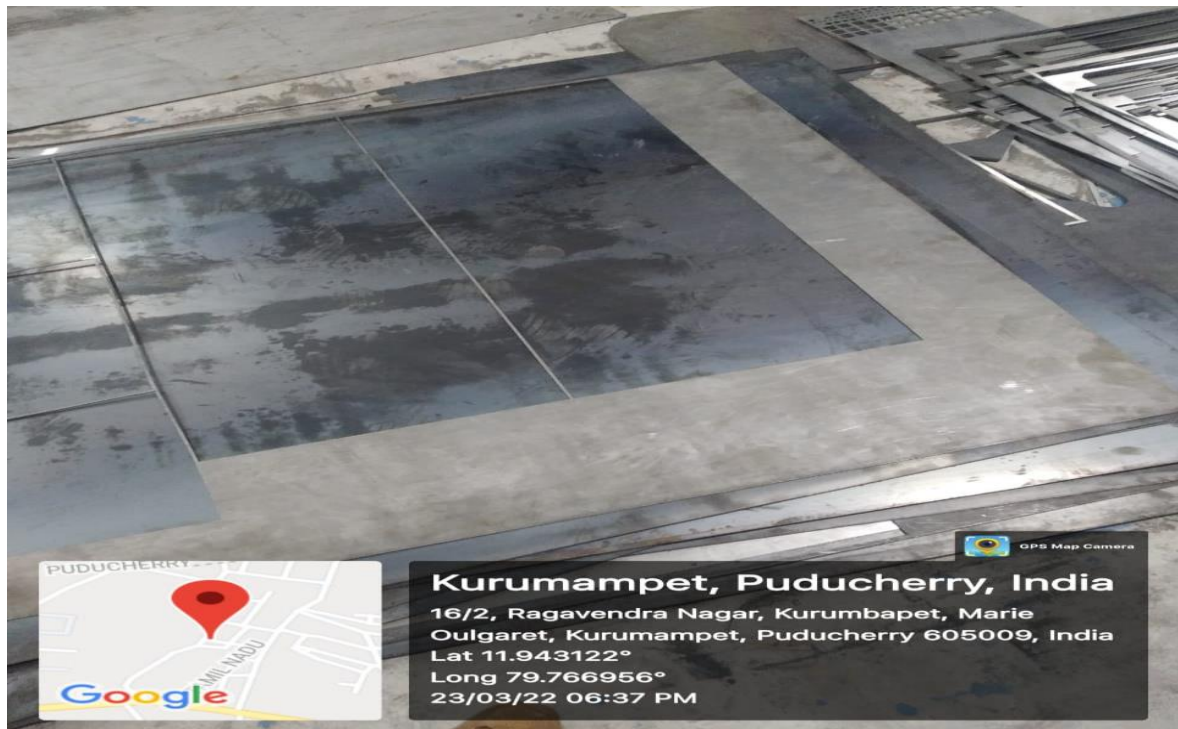
Fig 5.2 Marking for cutting sections
