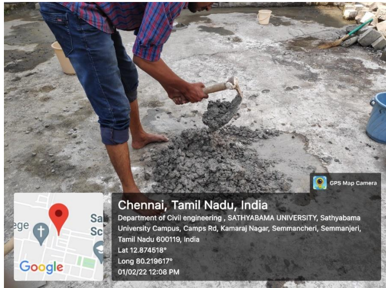
Fig.4.3 Concrete preparation
