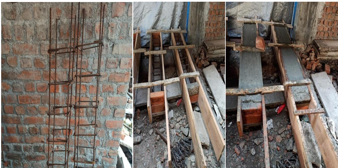
Fig.4.9 RC Beam Casting
