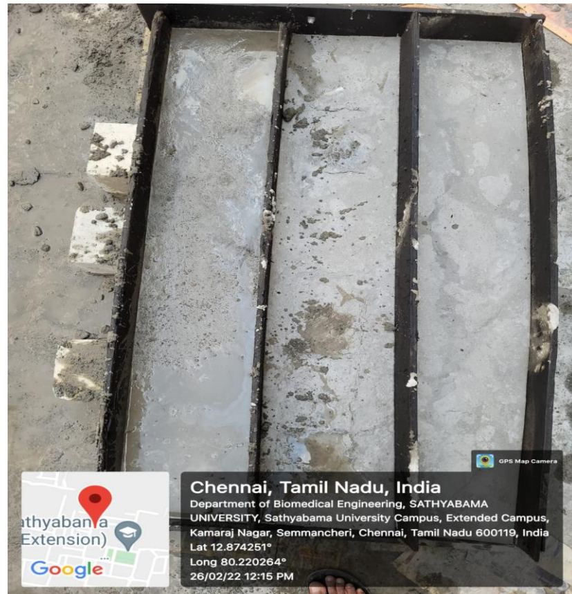
Fig.4.2. RC Beam Casting
