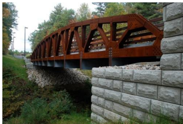
Fig. 1.2: An application of Corten steel bridge (source https://usbridge.com/ )
