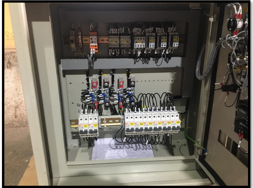
Fig 5.14: Logic panel components
