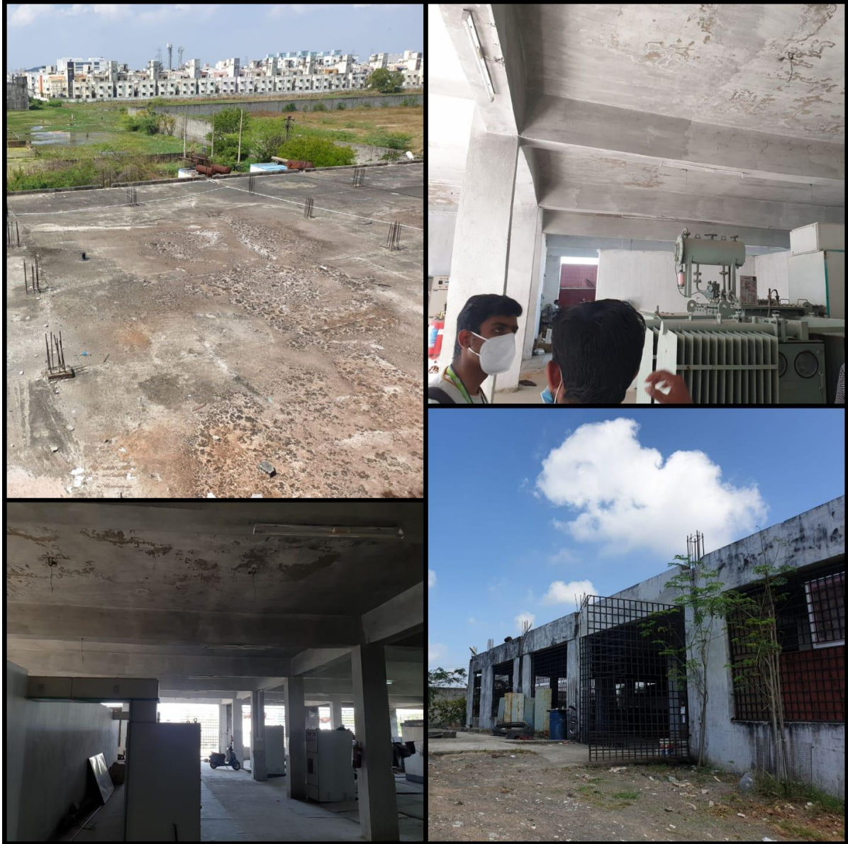
Fig: 3.1 First visit to Powerhouse-06.01.2022
