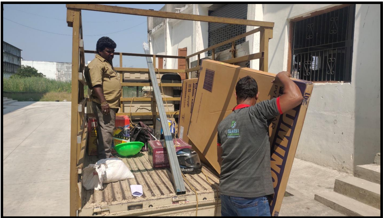
Fig 5.1: Unloading the Panels and components
