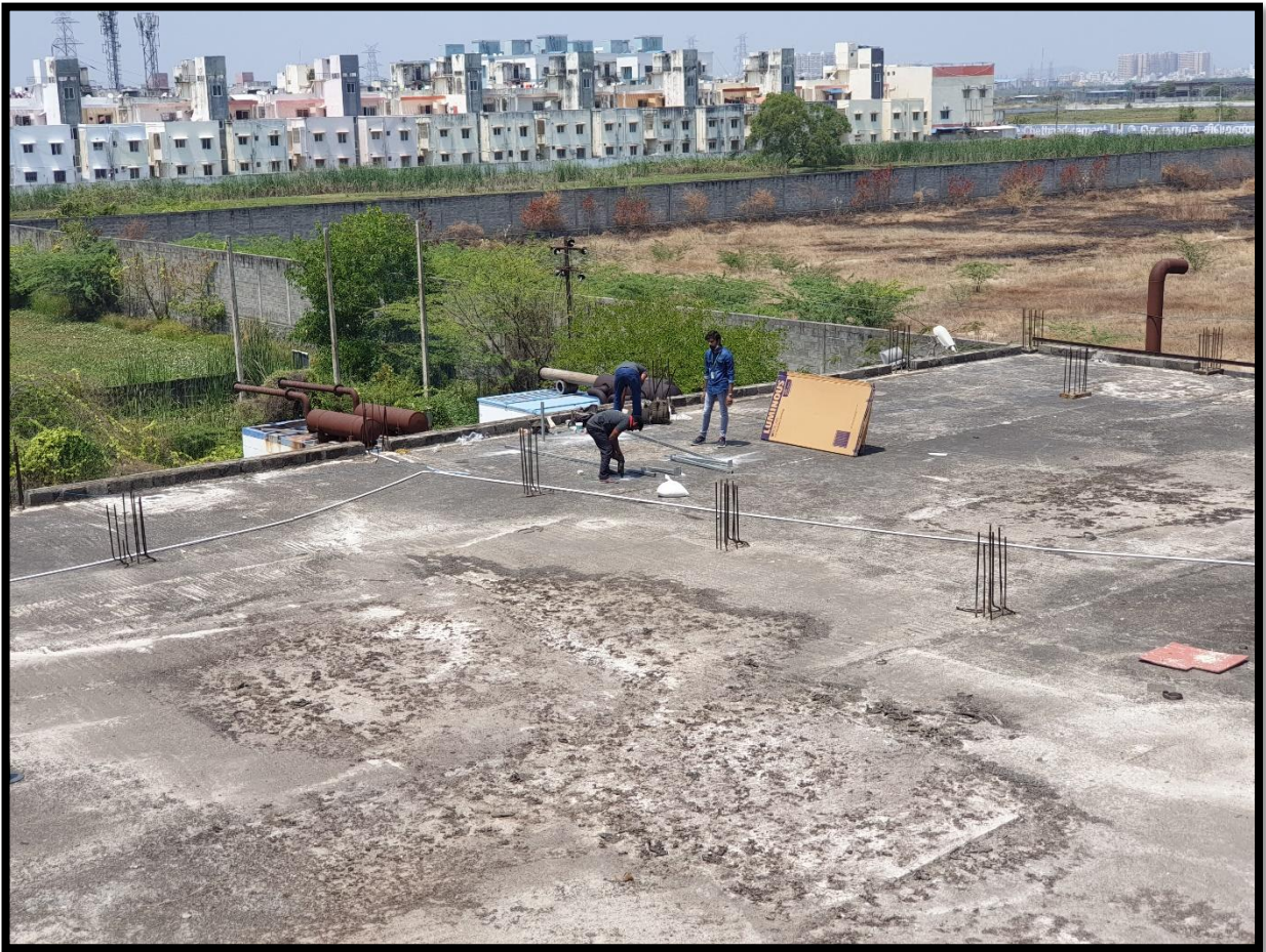
Fig 5.10: Mounting and Inspection
