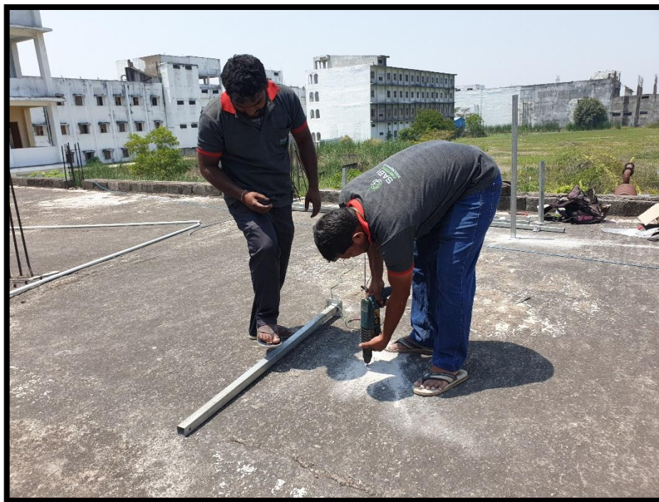
Fig: 5.3.: Drilling for Anchor fastening
