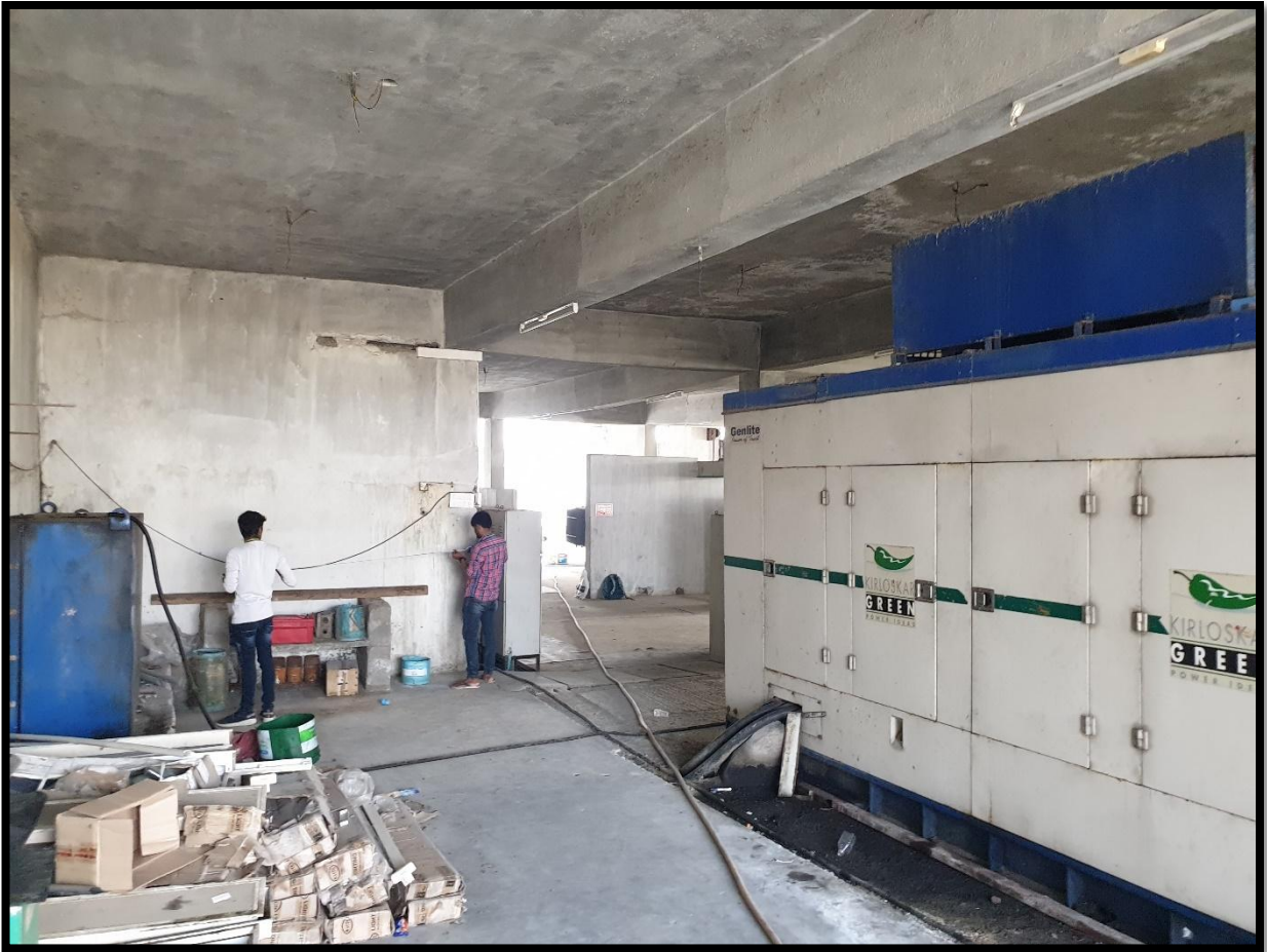
Fig 3.3 Mapping the powerhouse
