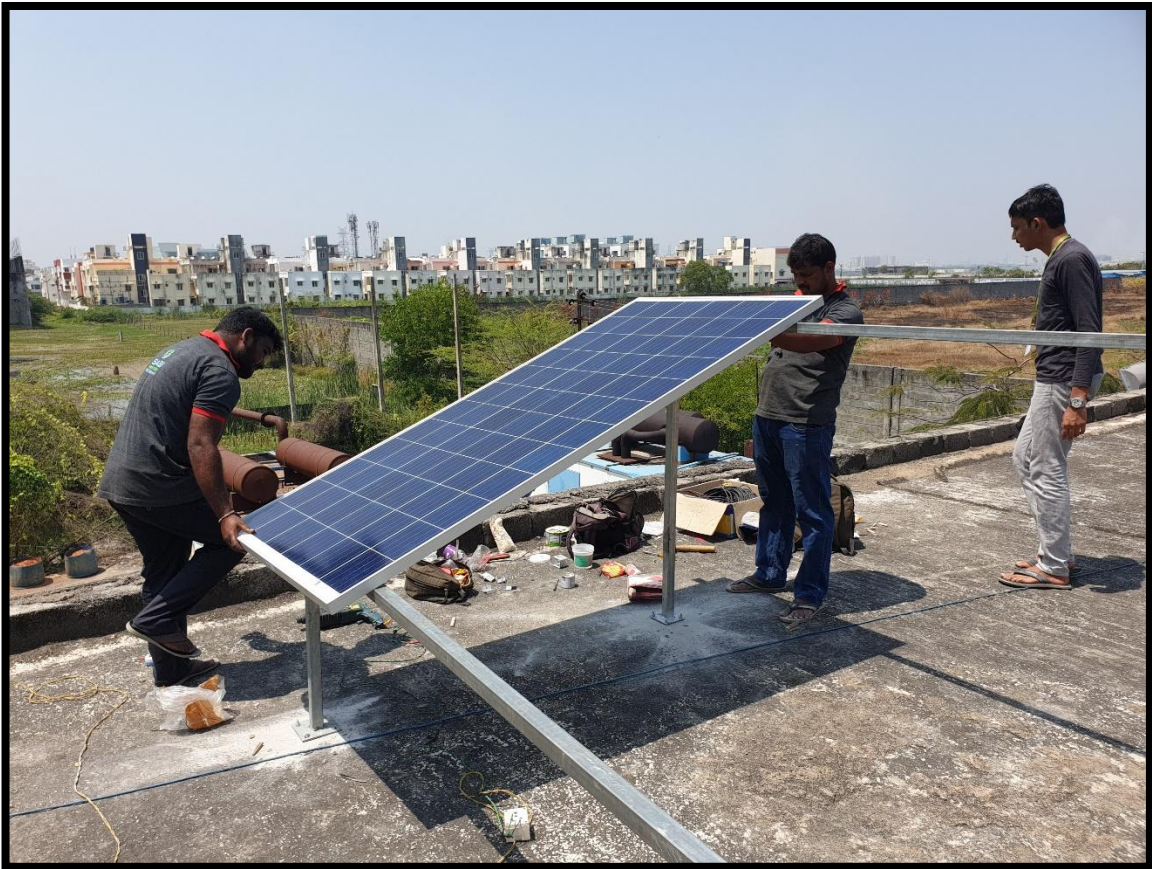
Fig 5.11: Panel Installation on powerhouse rooftop and inspection.
