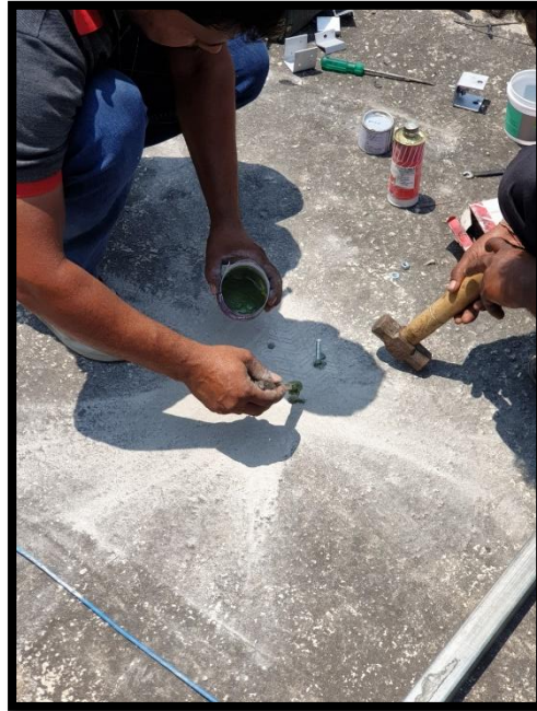
Fig 5.5: Chemical fixing
