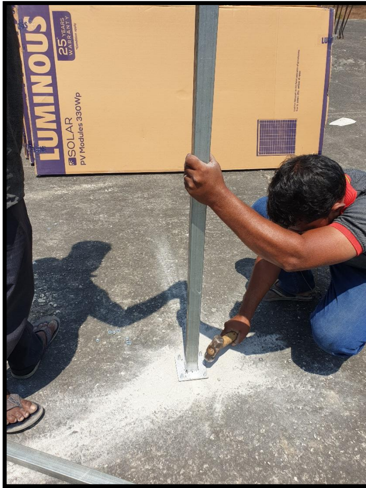
Fig 5.7: Technical team mounting the structure.
