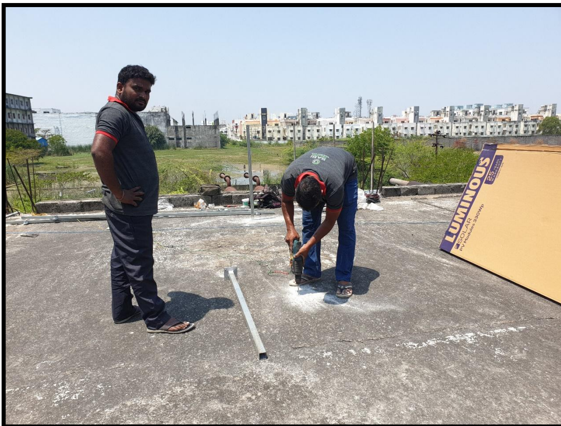
Fig: 5.2. Mounting the structure for solar panel (Technical team at work)
