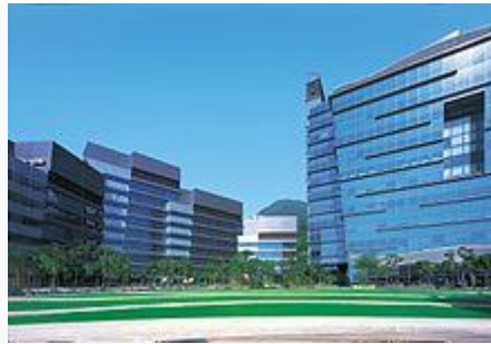
Figure 1.2 Hong Kong Cyberport 1 and Cyberport 2 Buildings
