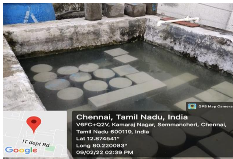
Fig: 4.6: Curing of concrete
