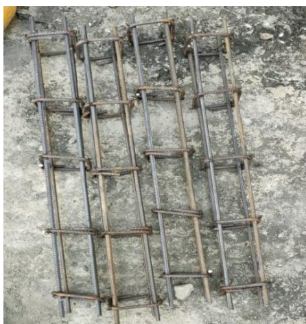
Fig:4.1 8mm reinforcement
