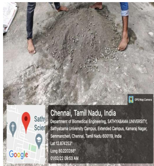
Fig 4.5 Picture of mixing concrete(Nominal Mix)
