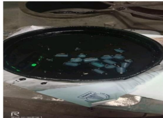
Fig: 4.2: Thermocol glue mixed with bitumen
