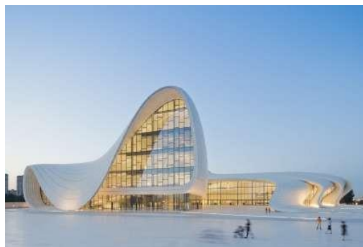
Fig 3.4.1 View of heydar aliye center
