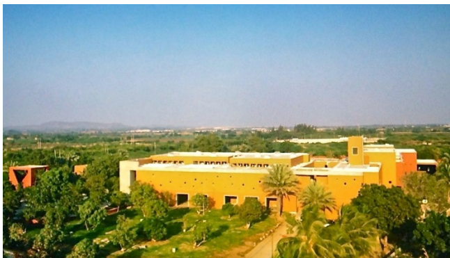
Figure 4.1 Exterior View of Museum Block
