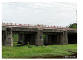
View into the site on the east
