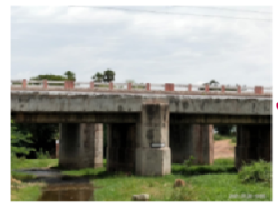
Gudur-Katpadi branch railway line
