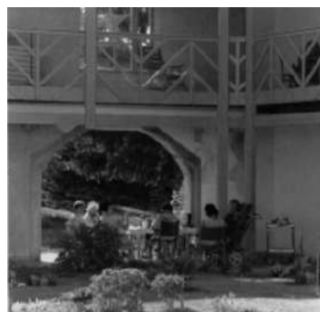
Fig 3.11 - The gallery arcade forms the natural boundary of the courtyard.
