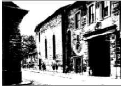
Fig. 3-3 : The facade provides an interface between the community and the health care facility and the external expression of the building's spirit within the community.
