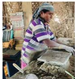
Step 5: Laying the wet mixture
