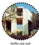
Waffle slab roof
