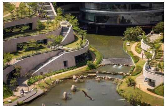
Fig.2.2 View of the existing lake extending into the structure.
