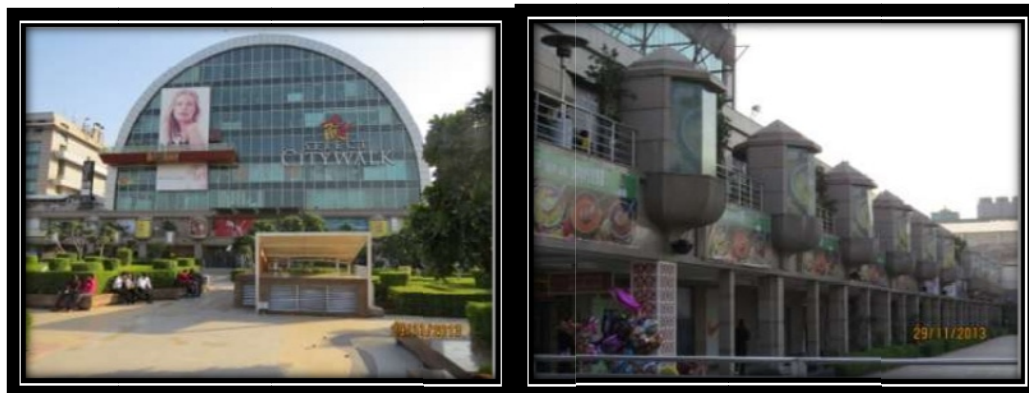
2.21 Select city walk external facades
