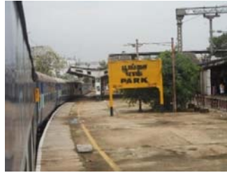
Figure 2.21 : Chennai Park Station
