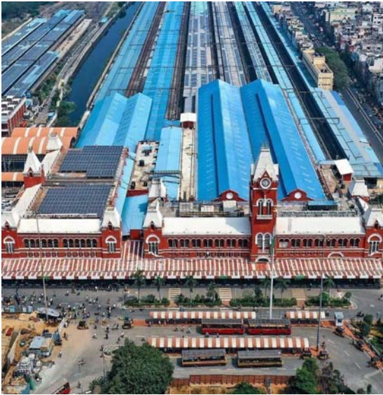
Figure 2.19 : Aerial shot of the Central
