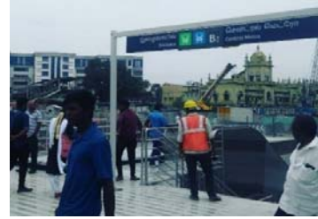
Figure 2.22 : Chennai Central Metro
