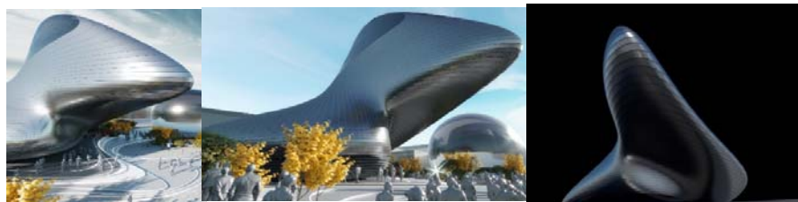
Fig 2.42 Façade view of the museum
