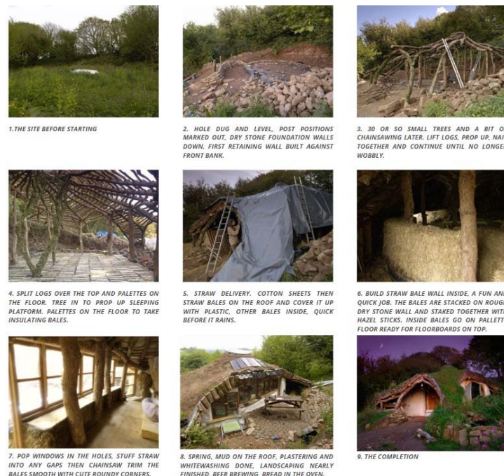
Fig 5.2 hobbit house construction phase
